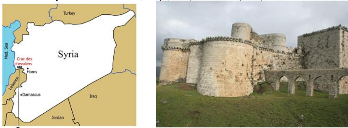
Figure 1 The location of Crac des Chevaliers on the Syrian map, with an overview of the southwest corner of the castle
